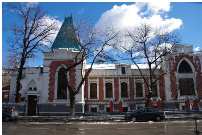
Fig. 1. Façade. State Central Theatre Museum "A.A. Bakhrushin", Moscow.
